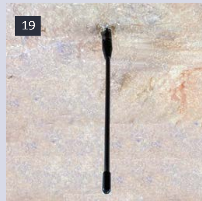
19: NCE RB02 through ceiling from below.
